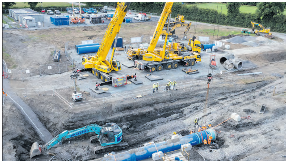
GOOD OPERATION: The works in Saggart Photos by Naoise Culhane
