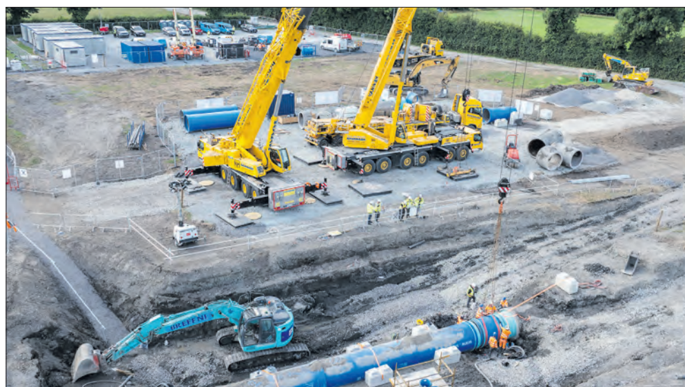
GOOD OPERATION: The works in Saggart Photos by Naoise Culhane
